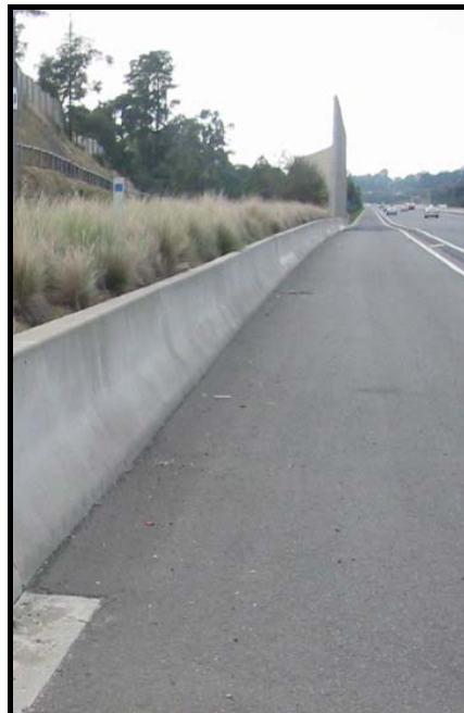
Concrete Barrier at Rear of the Left Shoulder on a Freeway
