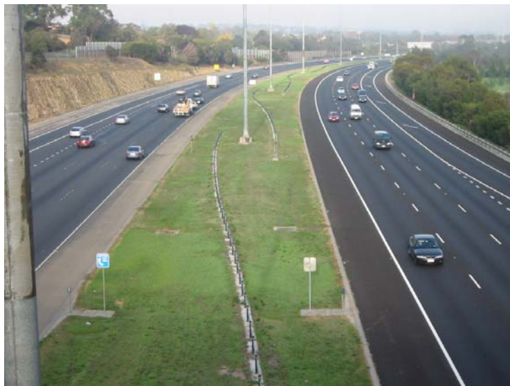
Wire Rope Safety Barrier in a Wide Flat Median
