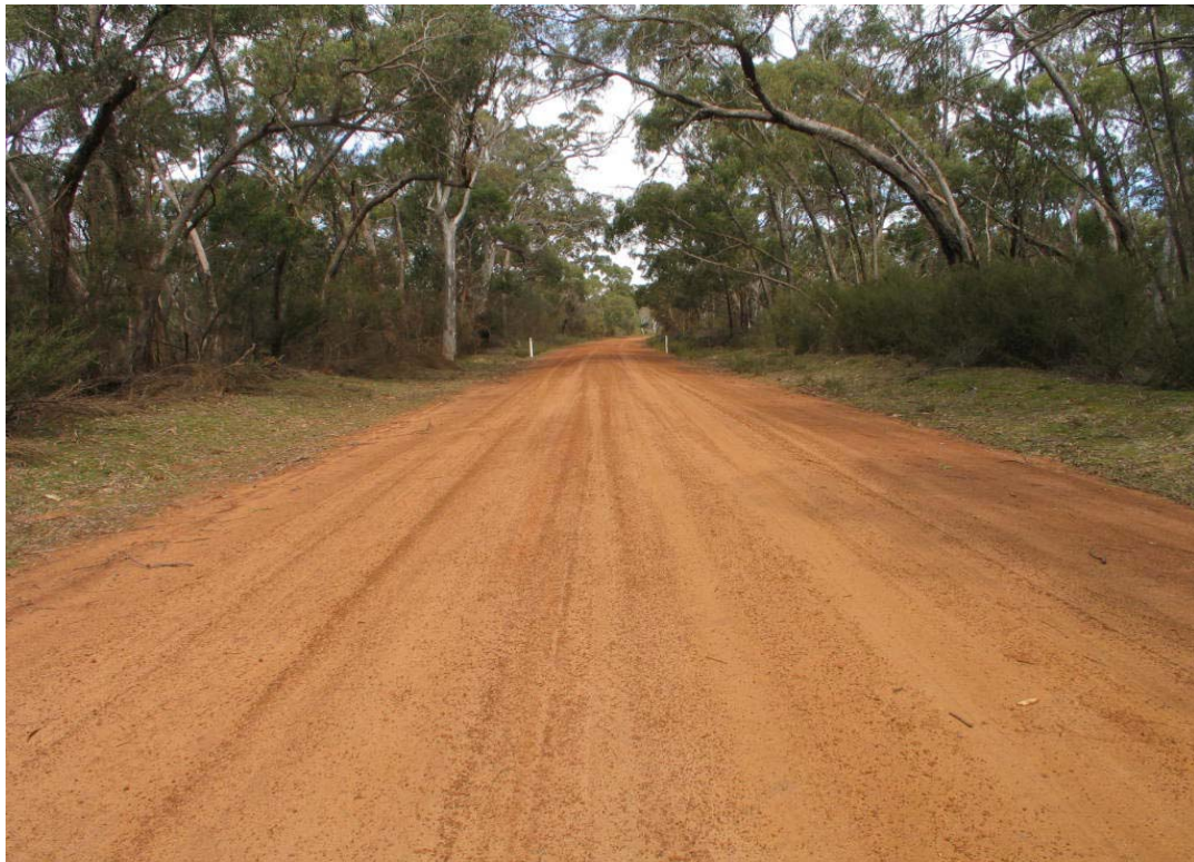
Figure 3.4 The image of a rural gravel road used in the survey
