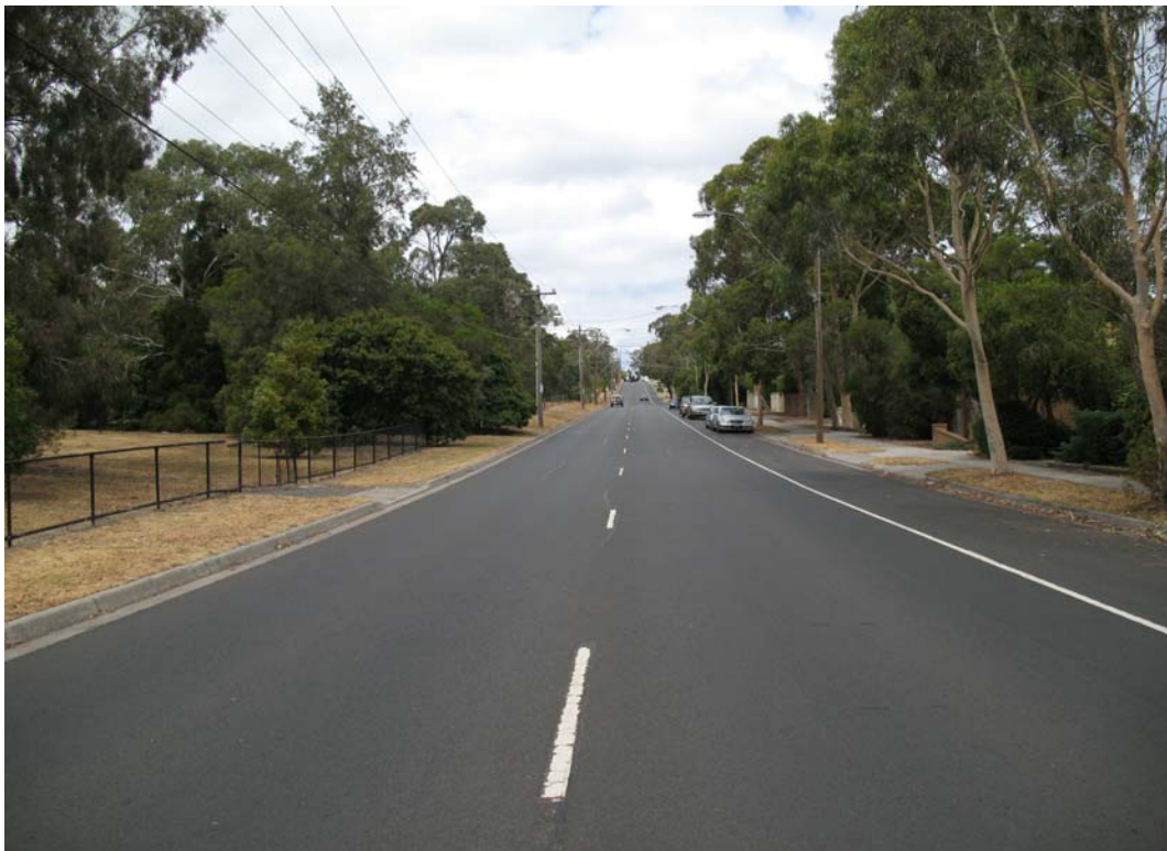
Figure 3.2 The image of a main undivided street in an urban area used in the survey
