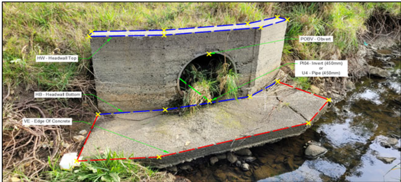
Example of Pipe Culvert inlet / outlet features
