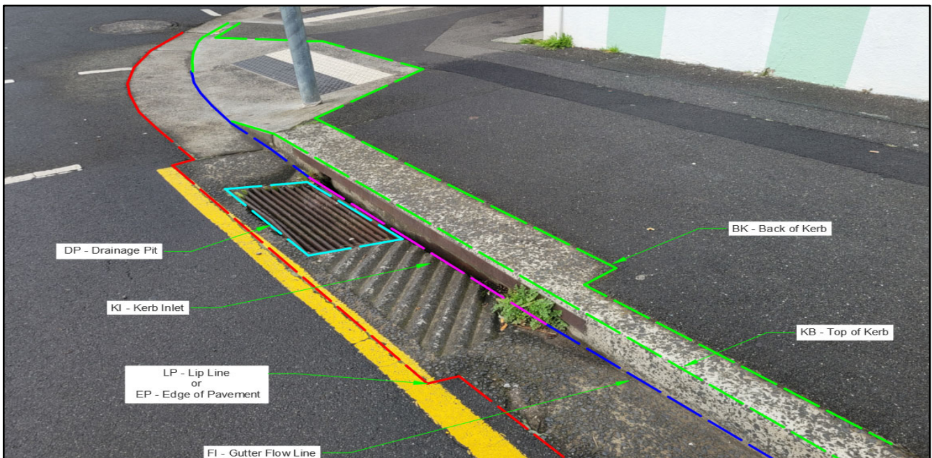
Example of Concrete Kerb and Drainage
